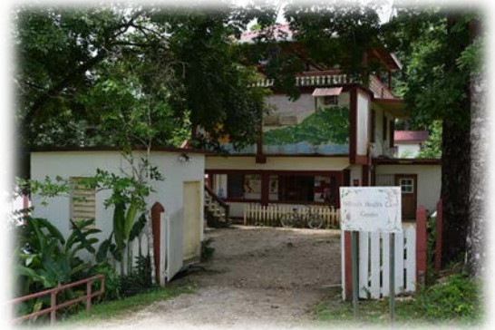
Outpatient Clinic at Hillside Health Care International Photo credit: Hillside website
